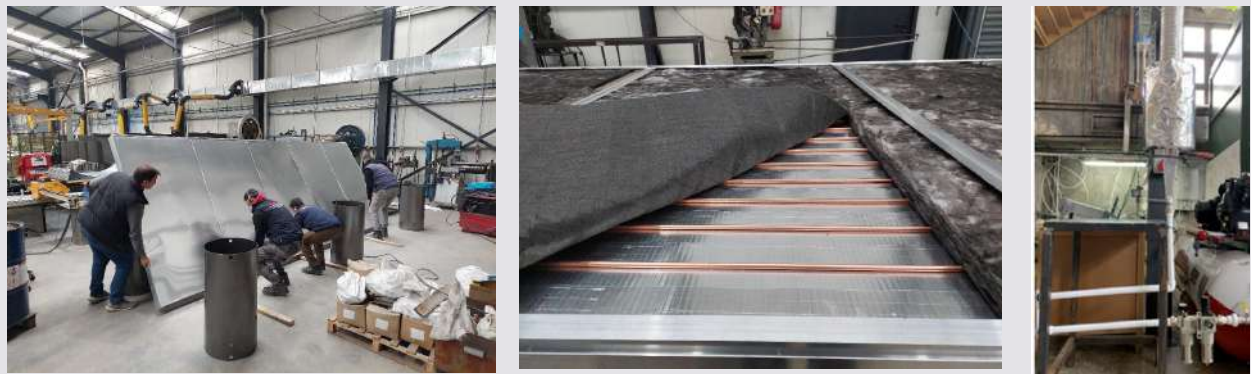
Figure 3: Solar thermal collector pilot construction phase & Laboratory test bed for the storage tank
