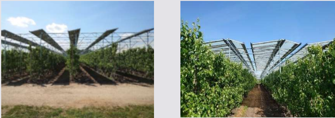
Figure 5: Photos of Agri-PV installations (BRITE)
